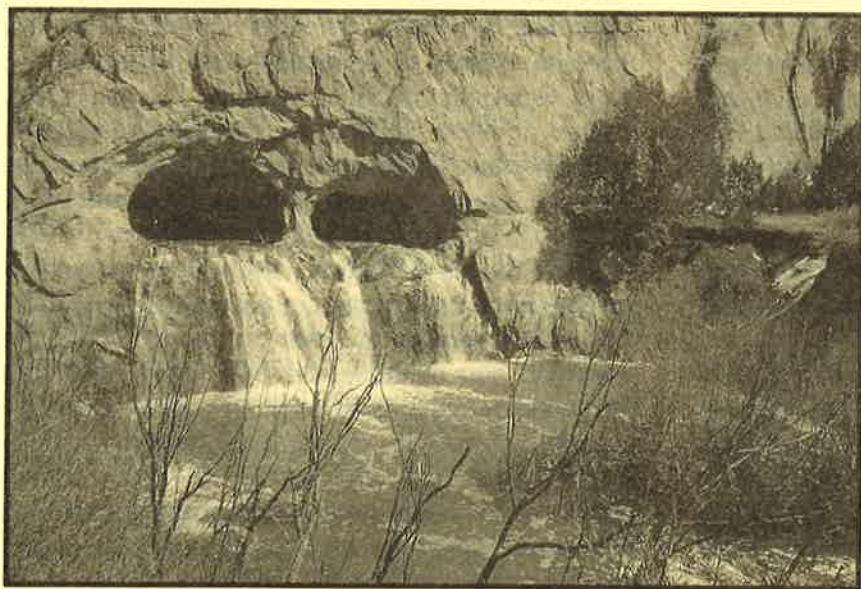
Spring floodwaters pass by the Nutria Irrigation District through the Upper Diversion Dam spillway. Note erosion in the fields on the left bank. Photo by D. Cleveland
