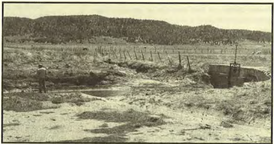
Lower diversion dam at Nutria in Spring 1993, before repairs started.
