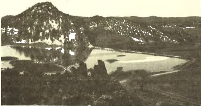
Nutria Diversion Dam and Reservoir. Excessive siltation over the years due to the poor condition of the upper watershed has greatly reduced the capacity of the reservoir. Photo by D. Cleveland
